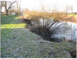
been stockpiled was closed down. I thought at the time that this was a false economy and a bad mistake. The flood tide rebounds from bank to bank as it progresses upstream and weak spots can develop, threatening the stability of the bank and the integrity of the flood defence. Periodic stoning in response to these events is the only answer.
